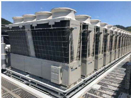
Module-type heat pump chiller (Minase Research Institute)
